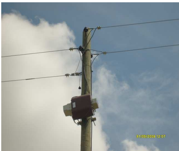
5. VROT-18-1 installed on pole
