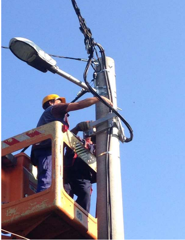
1. Console installation for VROT-18-3
