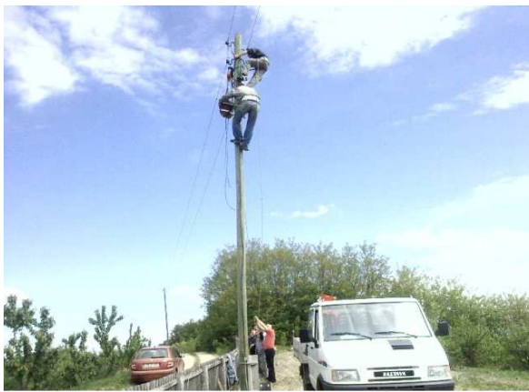
3. Lifting VROT-18-1 on pole
