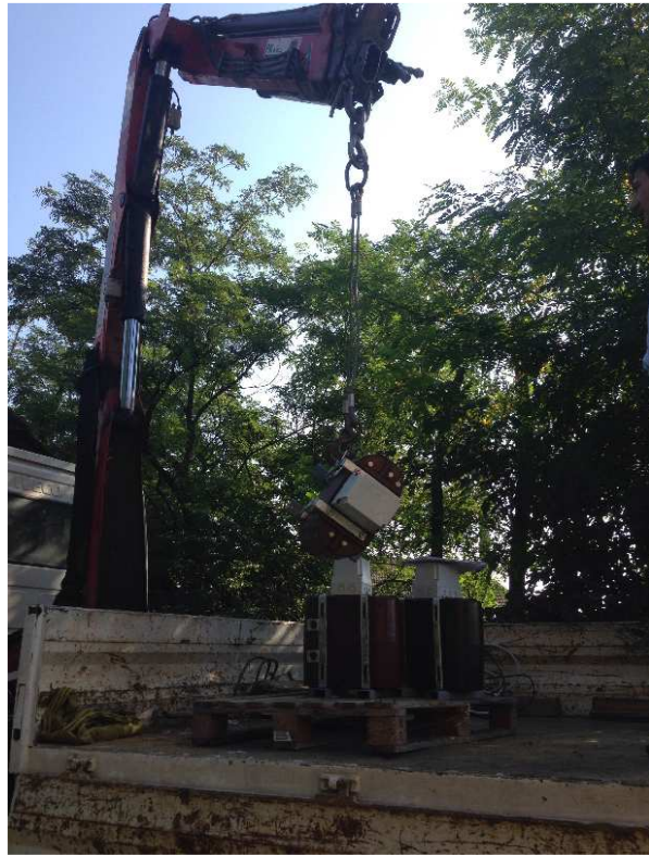
2. Lifting, VROT-18-3 on pole
