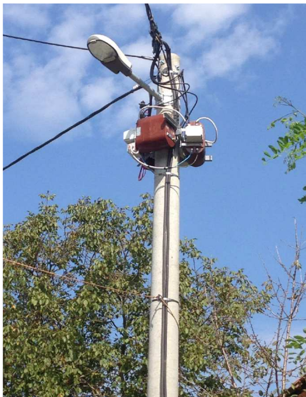
2. VROT-18-3 installed and energized
