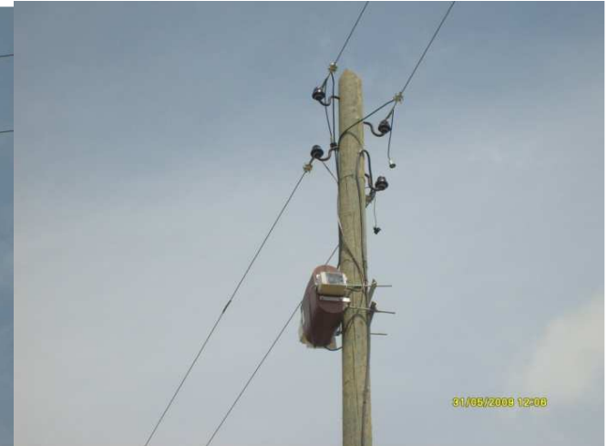
6. Atmospheric Lightning break surge arrester, VROT-18-1 is not damaged
